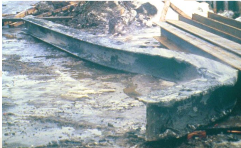
H-pile driven to sloping bedrock
