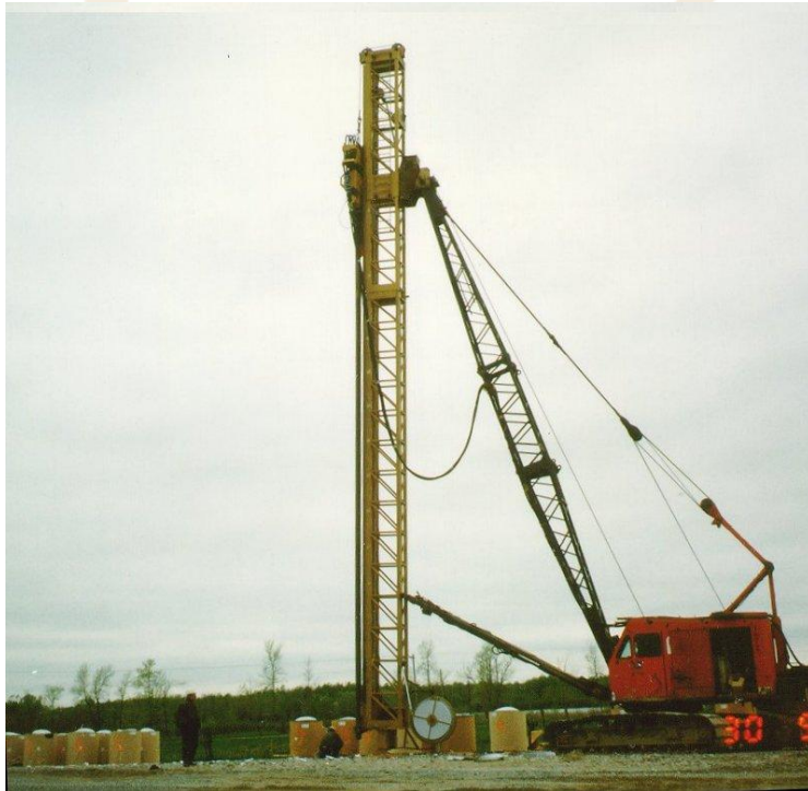
2000 HWY416, Ontario, wickdrain full-scale project
