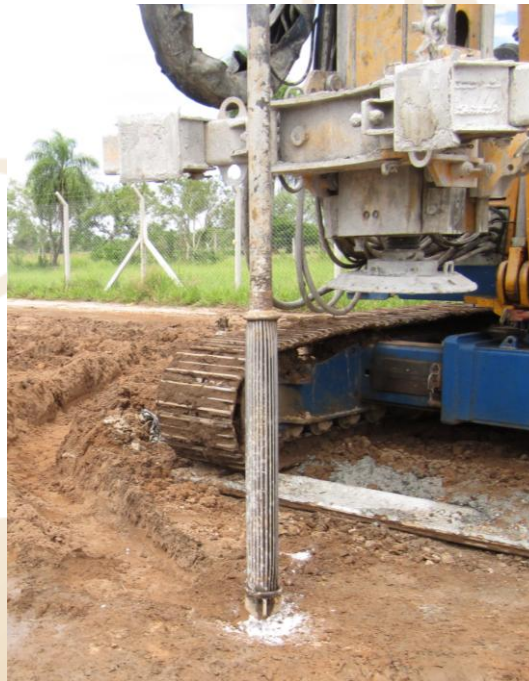
Installation of a pile with Expander Base (EB)
