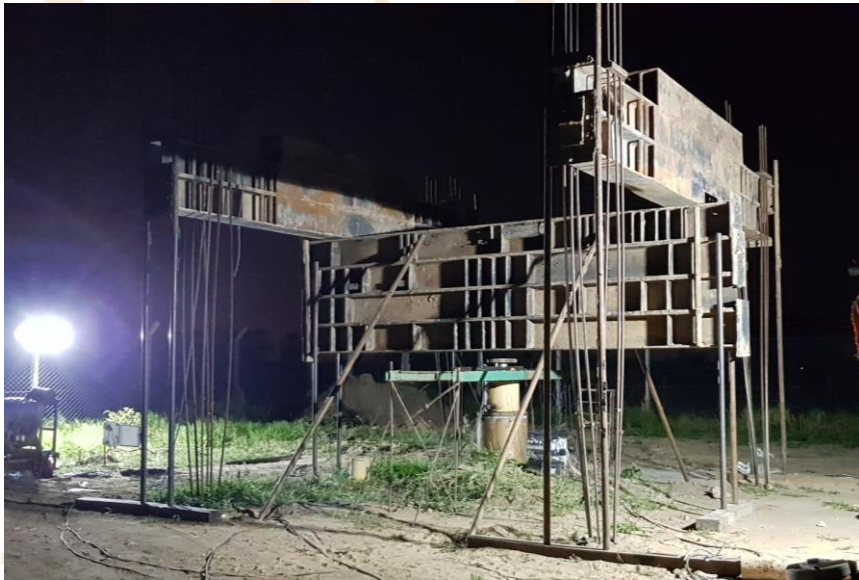
Ready for one of 25 loading tests.
