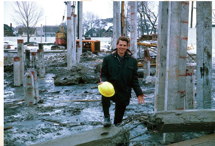
1974 Timmins, Ontario, resolving cause of broken piles
